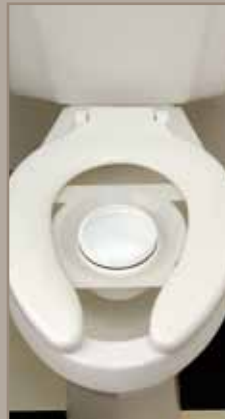
Figure 2. This top view of the toilet shows the toilet adapter holding the collection container in place. The toilet seat is down.
